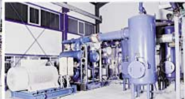
Multistage gas compressor
